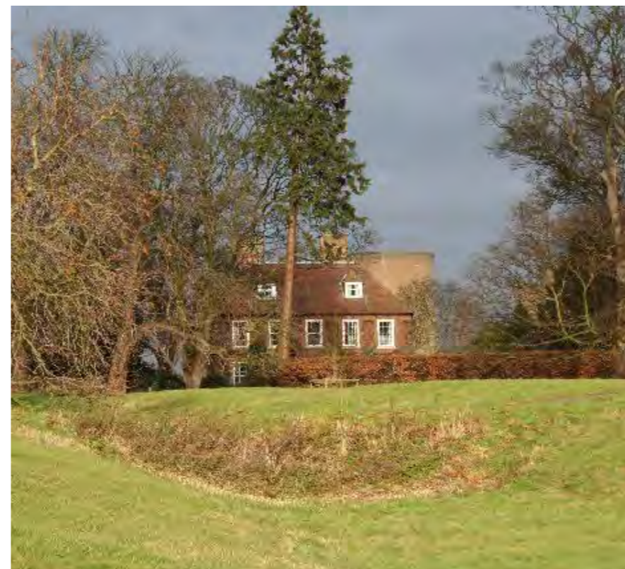
Photo of Asset, with now demolished cooling tower in background (Source: geography.org.uk)
