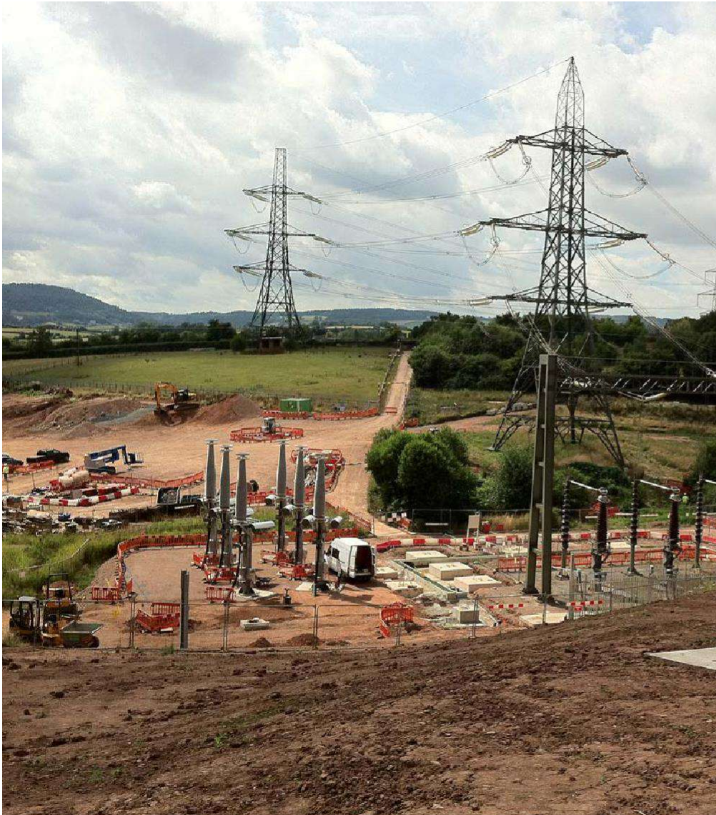
The undergrounding of electricity cables at Ross-on-Wye
